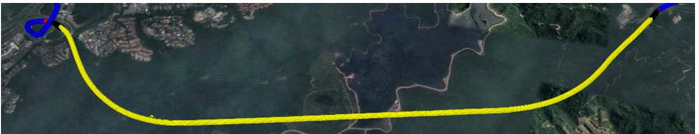
鸡公山隧道/Jigongshan Tunnel
